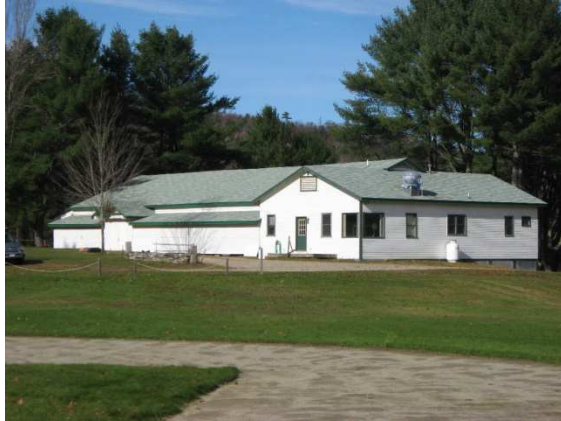
New Lodge roof
